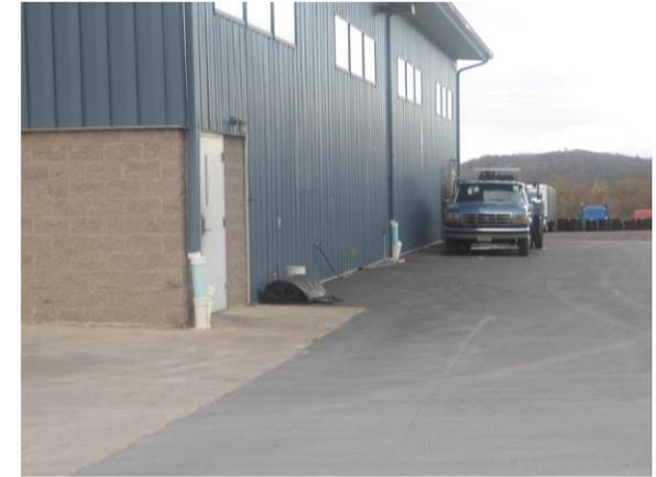
Parking spots can be replaced with porous asphalt to capture and infiltrate stormwater. Installing a cistern will capture roof runoff and provide water for washing vehicles or other non-potable uses. A preliminary soil assessment suggests that the soils have suitable drainage characteristics for green infrastructure.
