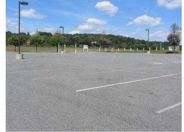
Parking spots of the site can be replaced with porous asphalt to capture and infiltrate stormwater. A preliminary soil assessment suggests that the soils have suitable drainage characteristics for green infrastructure.
