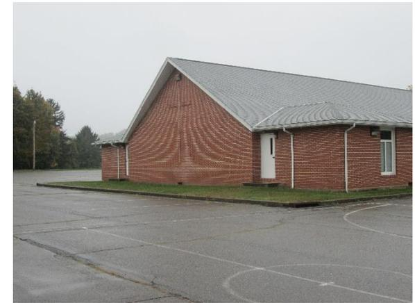
Rain gardens can be installed in front of the building to capture, treat, and infiltrate roof runoff. Runoff from the southeast corner of the building can be disconnected and rerouted into a rainwater harvesting system to be reused for watering plants. A preliminary soil assessment suggests that the soils have suitable drainage characteristics for green infrastructure.
