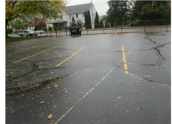
Parking spots to the south of the building can be replaced with porous asphalt to capture and infiltrate stormwater. Installing a rain garden adjacent to the building can capture, treat, and infiltrate roof runoff. A preliminary soil assessment suggests that the soils have suitable drainage characteristics for green infrastructure.
