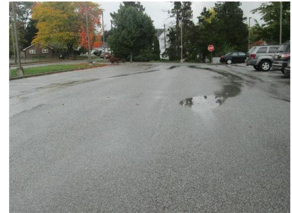
Parking spots in the west and south lots can be replaced with porous asphalt to capture and infiltrate stormwater. Installing a rain garden adjacent to the building can capture, treat, and infiltrate roof runoff. A preliminary soil assessment suggests that the soils have suitable drainage characteristics for green infrastructure.
