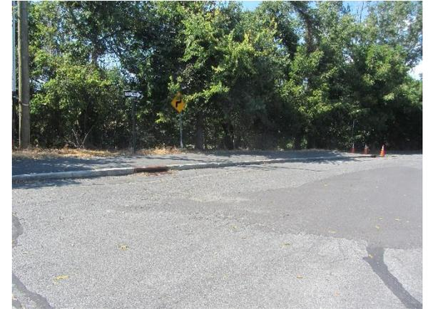
Parking spots along the western side of the lot can be replaced with porous asphalt to capture and infiltrate stormwater. Rain gardens adjacent to the building can capture, treat, and infiltrate roof runoff. A preliminary soil assessment suggests that the soils have suitable drainage characteristics for green infrastructure.
